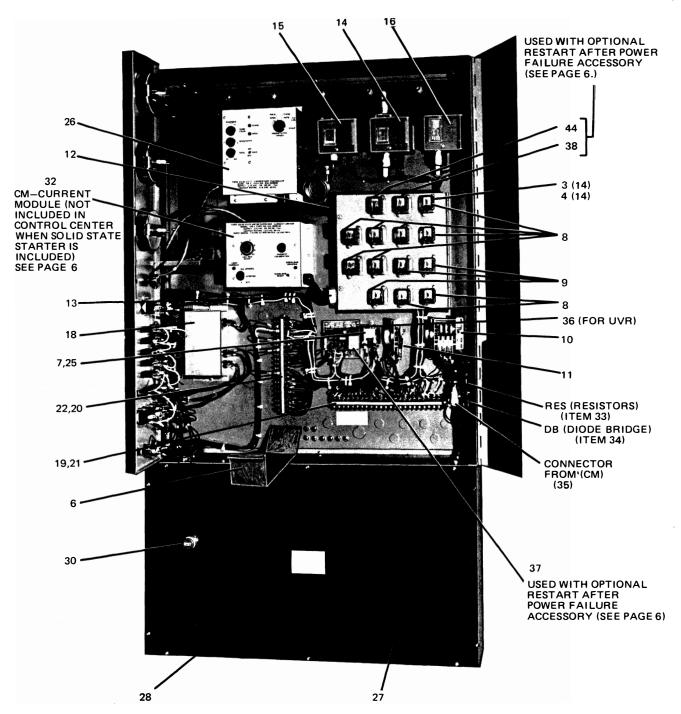
FIG. 3 - CONTROL CENTER - UPPER COMPARTMENT
